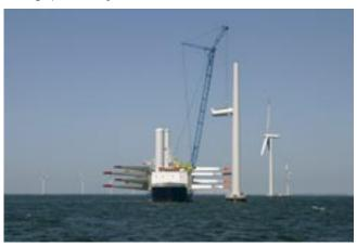
submarine, and Van Oord ACZ, an offshore sector construction and installation contractor. Other shareholders are Hovago Cranes (part of the Baris Group) and Marine Construct. The new company operates the purpose-built Jumping Jack (shown in Figure 5.8), a jack-up barge with an onboard crane, which was used to install the Horns Rev foundations.
